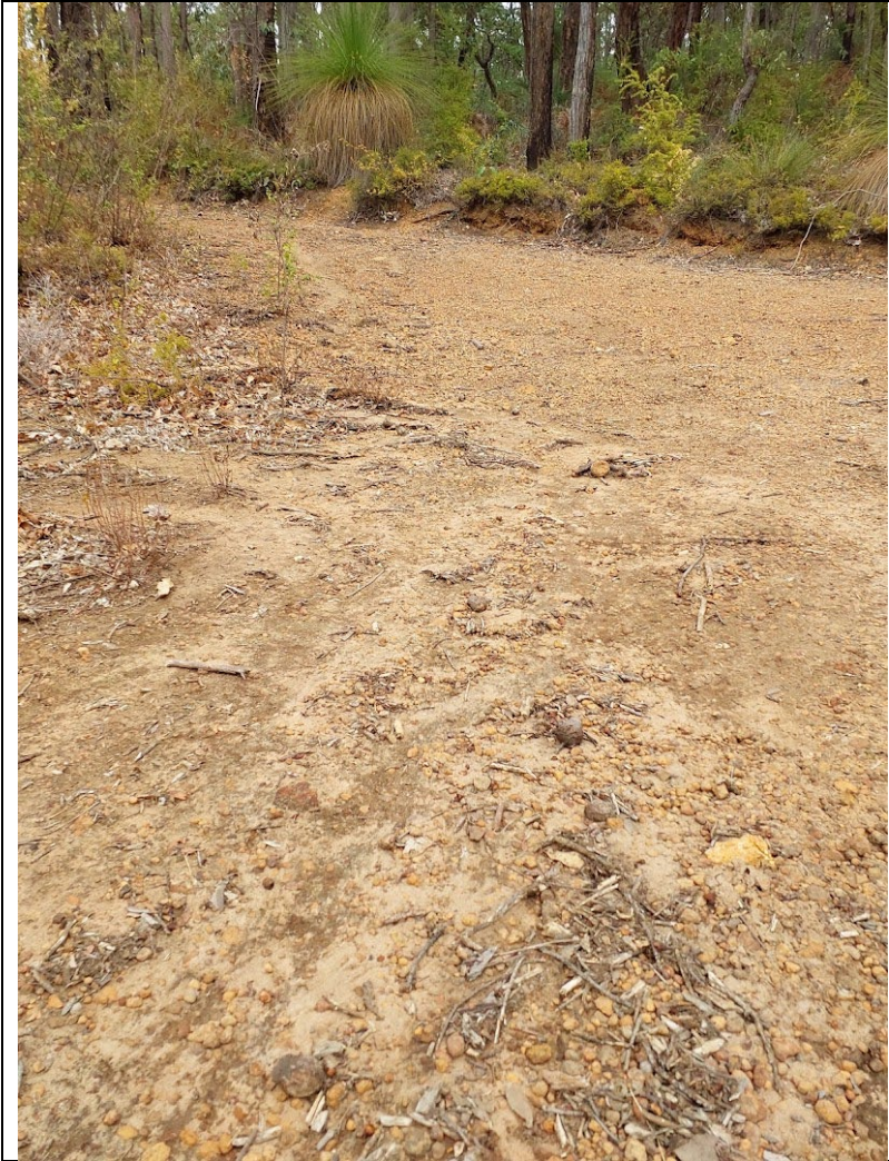
Bush track to PD01 – slight water erosion lines observed
