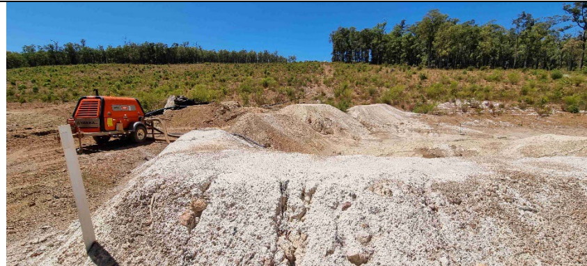
Marshall 13: sump with pump to transfer water to other side of catchment if required.
