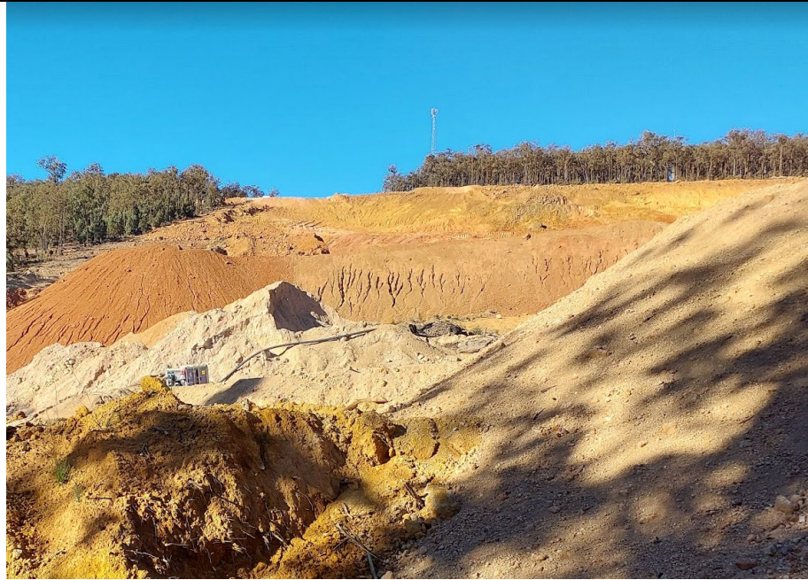
Fresh clay moved for drainage control at Mabbott 1
