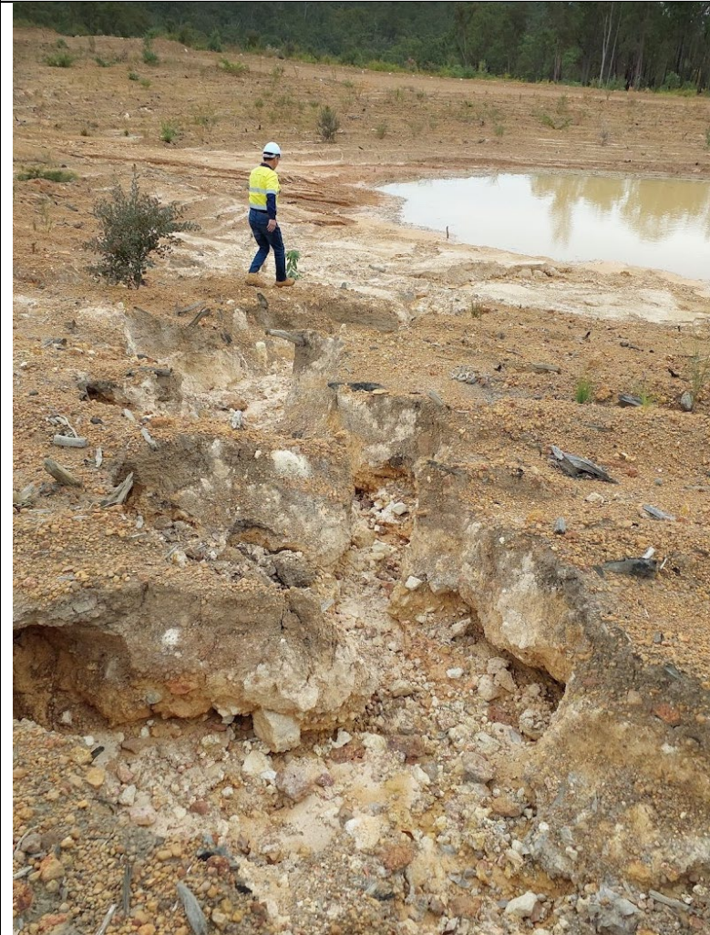
Another erosion area at Dellamaddalena 5
