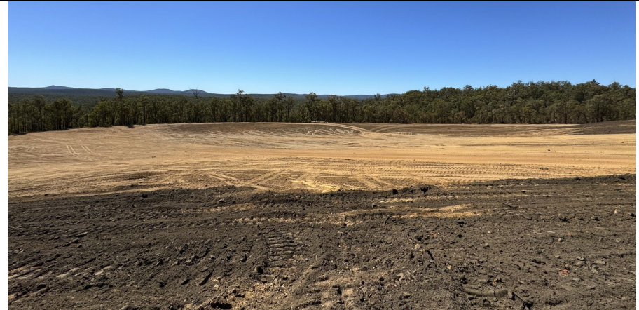
Topsoil return at Rance 5. This area is within the 1km dam top water level zone and about 350 m to the nearest stream.
