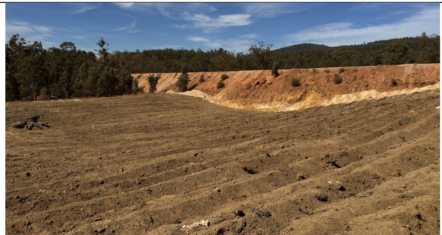
Walk track around disturbed areas at Kisler 13 (left). The bottom of the pit is rehabilitated with drainage controls (contour ripping and drainage control sump) in place (right).
