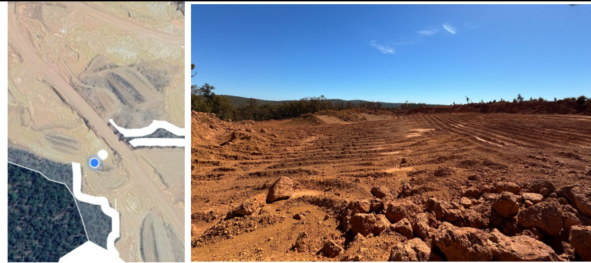
Newly ripped pit floor for stabilisation at Gibber 15
