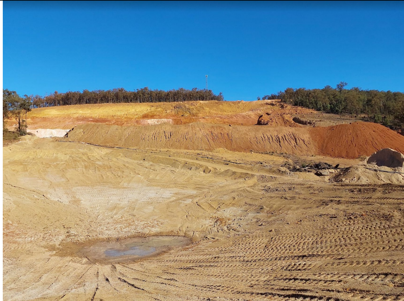
Drainage basin at Mabbott 1
