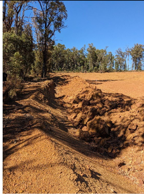
Gibber 15 – pit is sloped towards road and away from forested areas. Bund also to prevent water entering forested area to the left.
