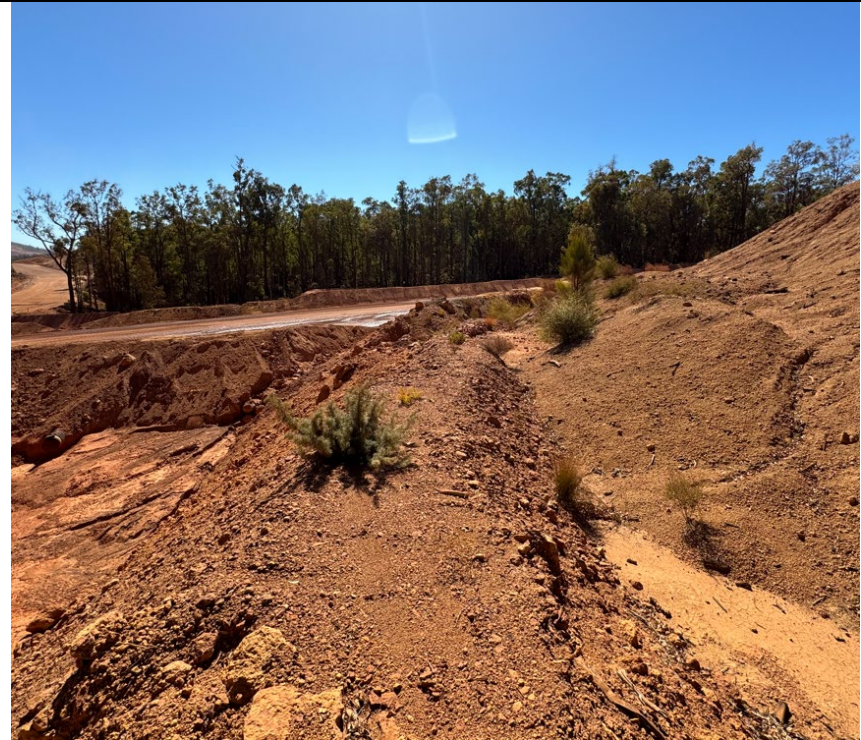
Downes 8 drainage risk area. Storm water from this area reports to road sump (right). This area is currently assessed as high drainage risk area.
