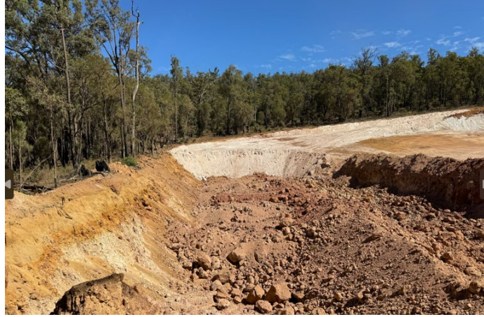
Eastern pit boundary and drainage control feature at Stone 6.
