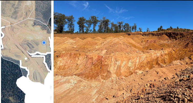
Newly cut trenches at Gibber 15 for drainage control
