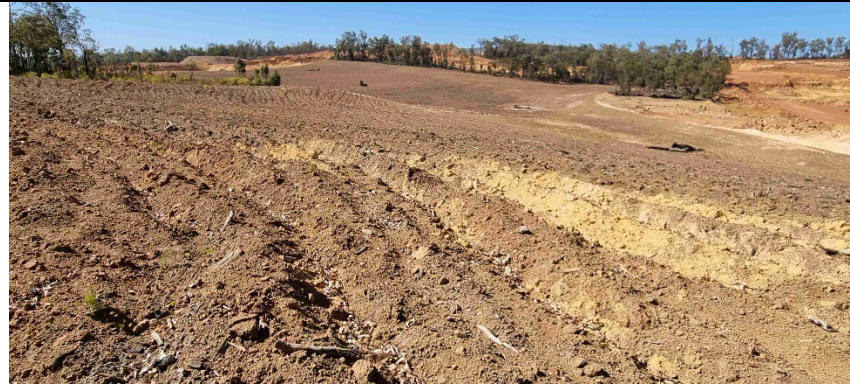
Rance 6: compartmentalised catchments, ripping on contour, basins installed in rehabbed areas.
