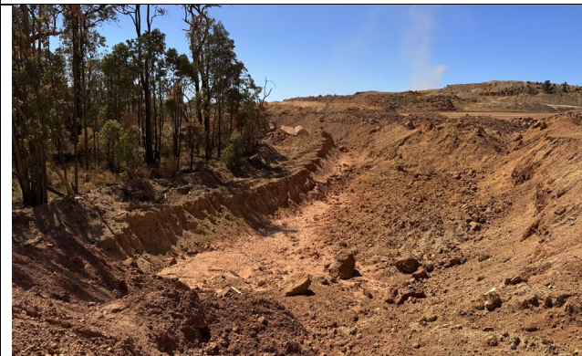
Interim drainage control at Kisler 11. Cut volume to catchment volume ratio is between 25-50% in this area.
