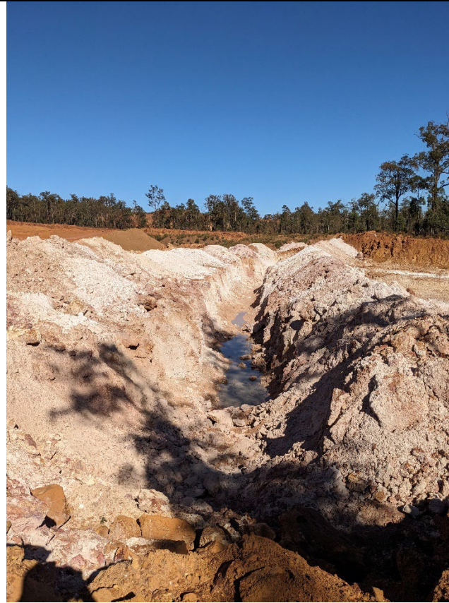
Gibber 16 – recently completed trench made of clay with groundwater present.
