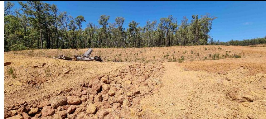
Marshall 14: basin installed in rehab, with rocky spillway for controlled release of water if basin capacity is exceeded
