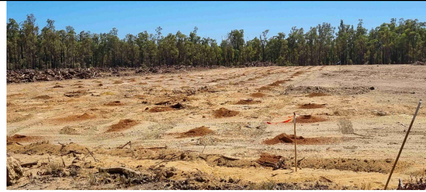
Wittwer-11: water shots (although not yet blasted) to promote infiltration
