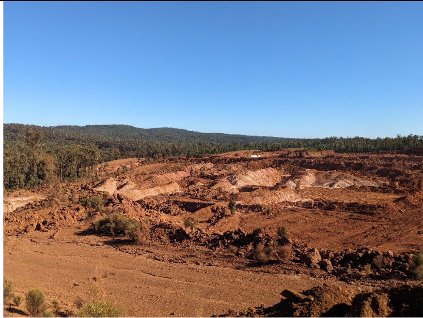
Gibber 12 – trenches sumps, and stockpiles at Gibber 12 .
