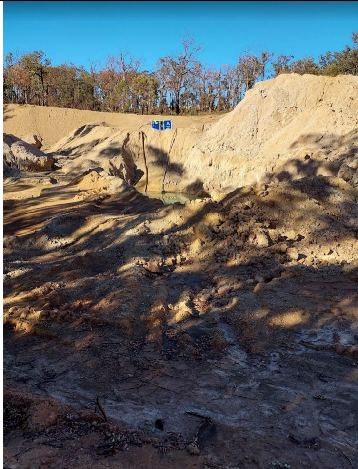
Trench with Pump at Mabbott 1
