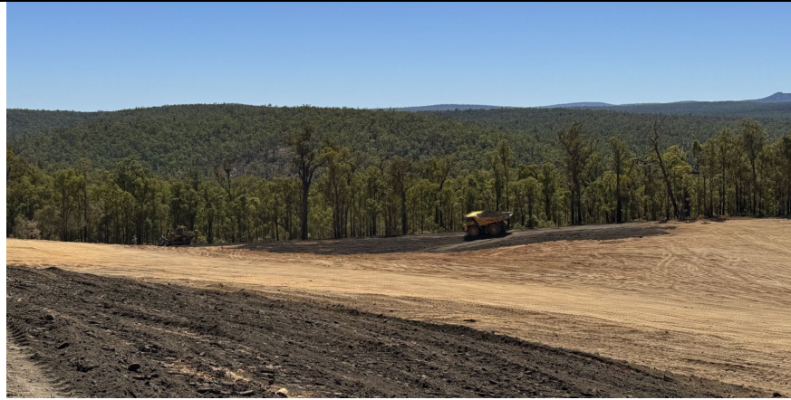
Topsoil return at Rance 5. This area is within the 1km dam top water level zone and about 350 m to the nearest stream.
