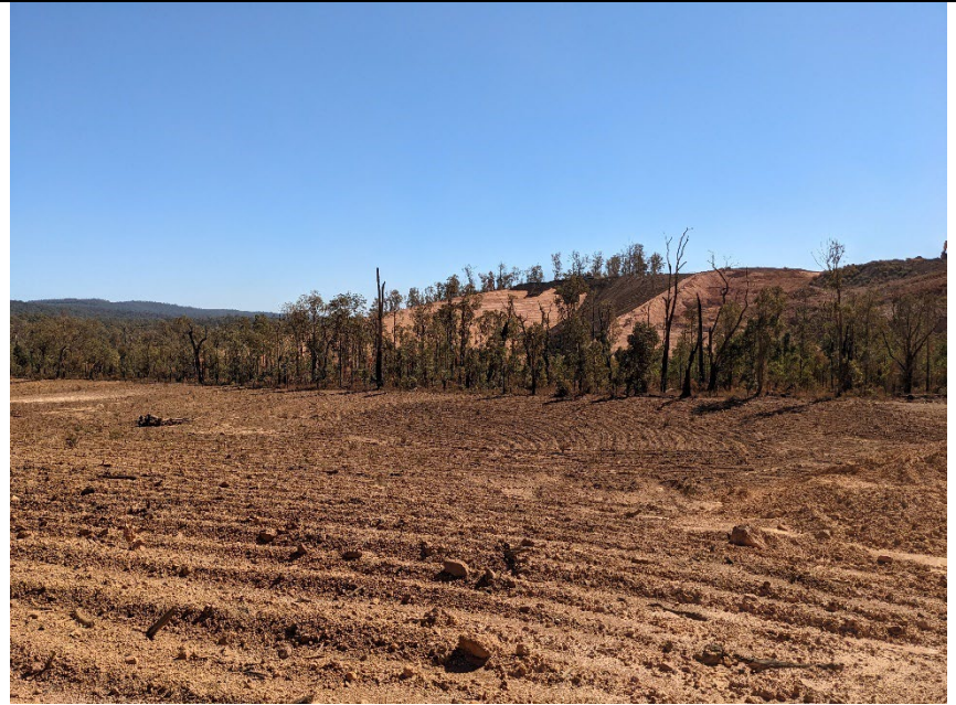
Vaquita 8 – contour ripping and bowls at Vaquita 8.
