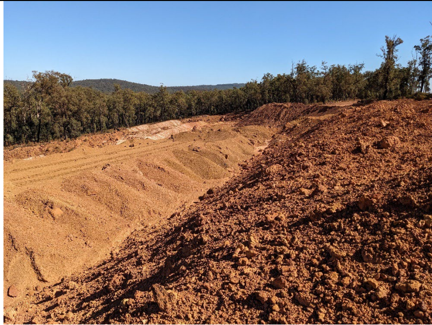
Minke 3 – trenches observed
