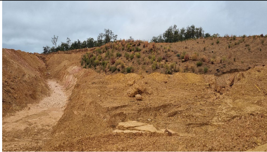
Rance 1 trench leading to sump segregating rehabilitated area from dieback stockpile.
