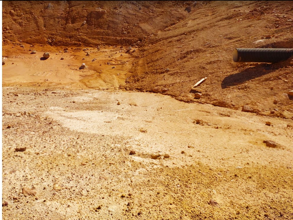
Drainage sump at davey 1
