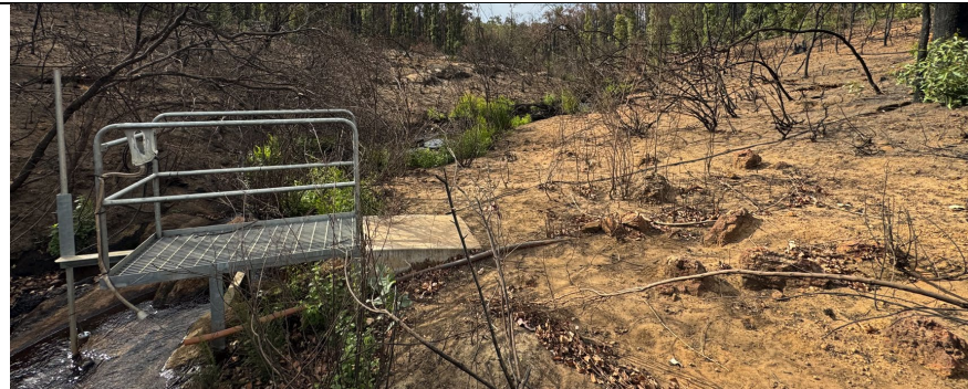
Burnt state of the vegetation cover around turbidity monitor SE59.
